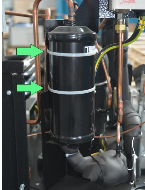
Fig. 19 - Ties holding filter-receiver
