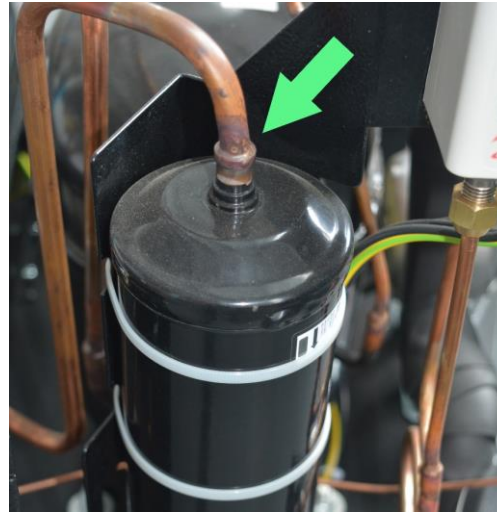
Fig. 17 - Top receiver - filter tube
